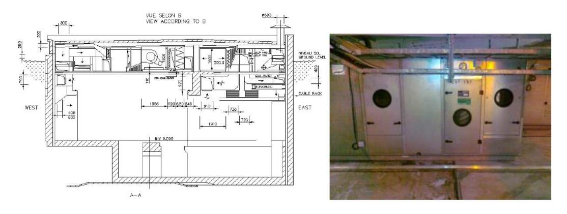
Linac3 – Ventilation is insufficient to properly operate Linac3 to design spec, the asbestos in the ceiling needs to be dealt with at the same time.
