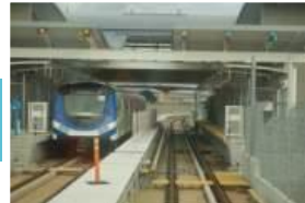
Rail signalling systems
