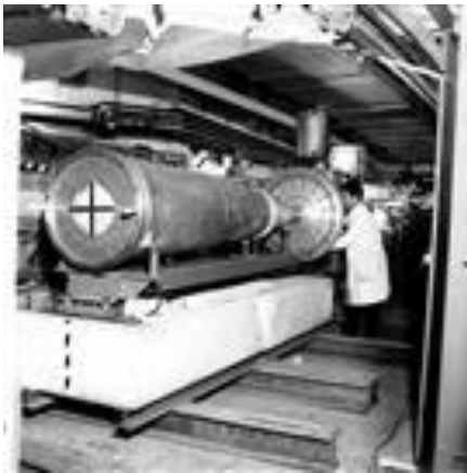
Horn installed on the beam line (1964)
