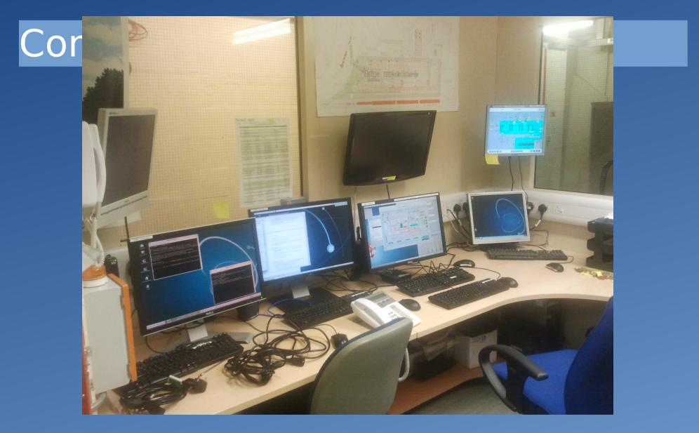
3 seating positions - shorter desks and remove curved section Double HD monitors at each desk (1920 x 1200) Large monitor/TV on Wall for alarm handler and other status information
