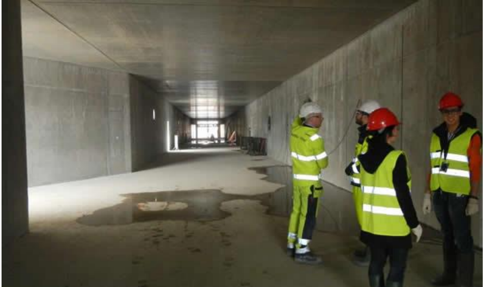
Accelerator tunnel at ESS, Lund, Sweden
