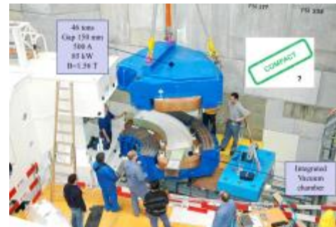
Gantry, 90 deg dipole w/ integrated vac chamber
