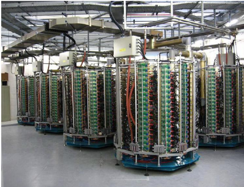
SOLEIL 45 kW @ 352 MHz solid state amplifier towers (2004 & 2007)
