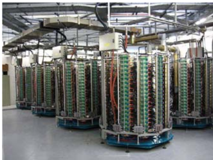
SOLEIL 45 kW @ 352 MHz solid state amplifier towers (2004 & 2007)
