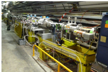
UA9 installation in the SPS
