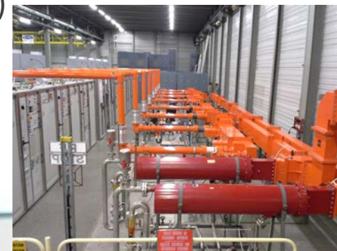
SPS IOT 801 MHz 2x240 kW CW
