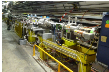
UA9 installation in the SPS
