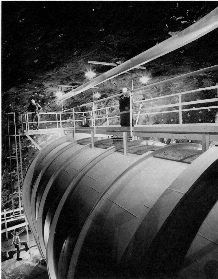
Davis' neutrino detection apparatus one kilometer underground in the Homestake Gold Mine, Lead, South Dakota. The tank contains 400,000 liters of perchloroethylene.
