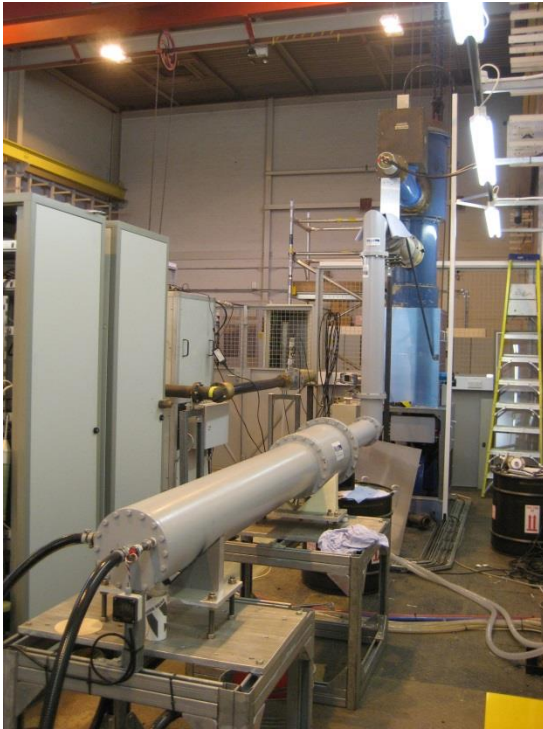
RF System in Plant Room 1
