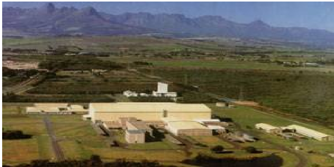
Isotope Production, Medical Irradiation, Education and Training, Research. 3 accelerators (K200 cyclotron, 11 MeV cyclotron and 3MV van de Graaf for Materials Research)
