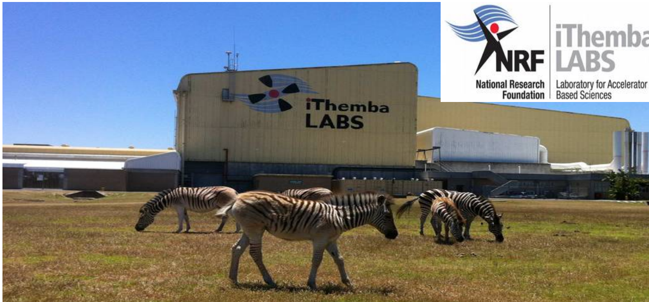
Largest Science Facility in the Southern Hemisphere (a place of Hope)
