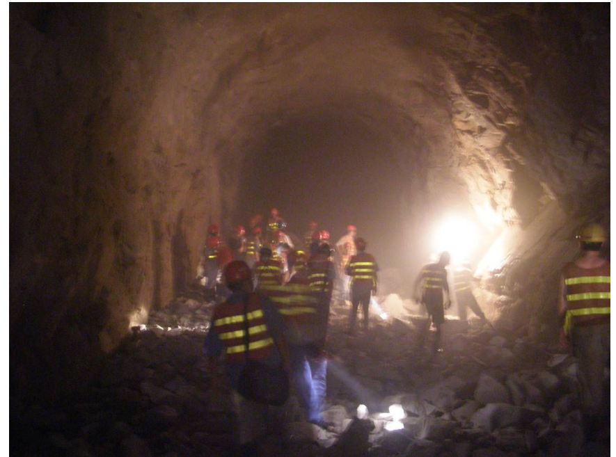
Main Tunnels Join - June 09
