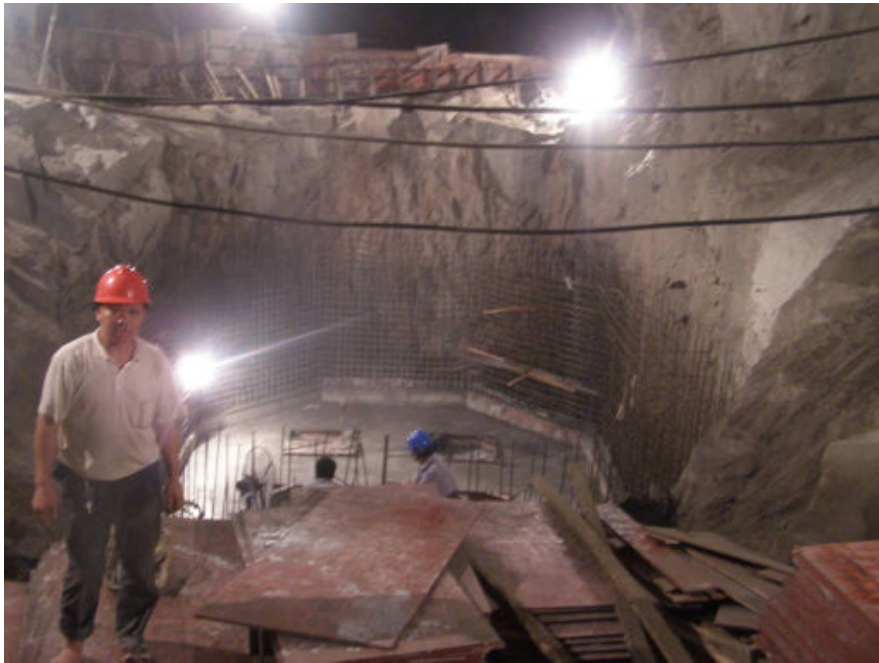
Pool Excavation in DBY Hall - Aug 09
