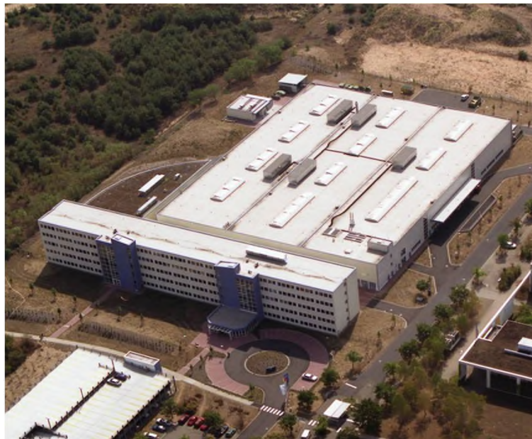
Bruker HTS plant in Alzenau, Germany
