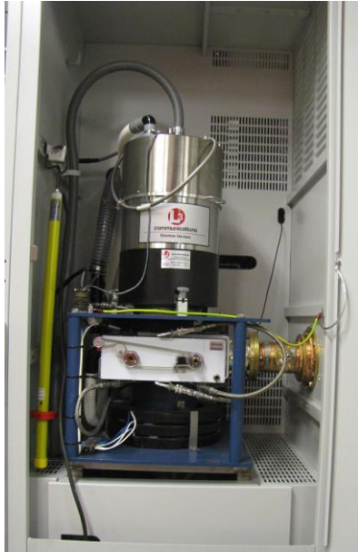
Elettra 500 MHz 150 kW IOT based amplifier for Combination of 2x80 kW
