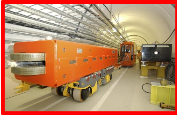
CERN LHC conventional-magnet installation Capacity: 9 t per buggy Eq. height: 560 mm
