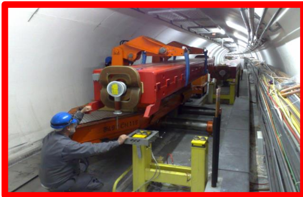
CERN SPS conventional-magnet installation Capacity: 20 t Eq. height: 800 mm
