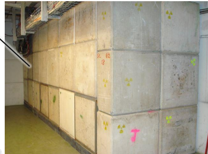
Additional shielding on primary area side
