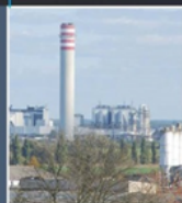
Controlling power plant
