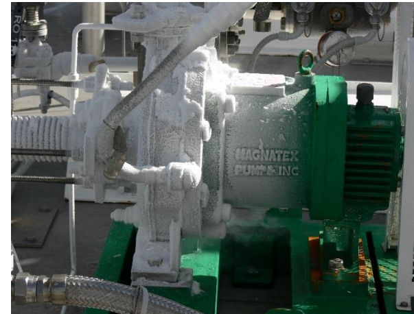
Magnetic Coupled Cryogenic Pump
