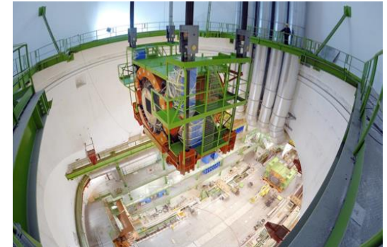
Mechanics for forward hadron calorimeter
