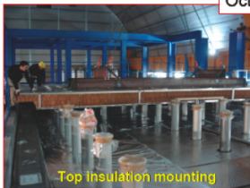
Top insulation mounting
