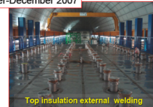
Top insulation external welding
