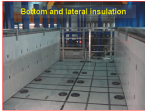
T300 modules in position
