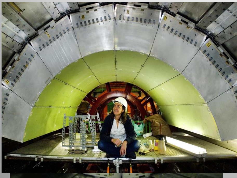
Central ECAL installation in CMS
