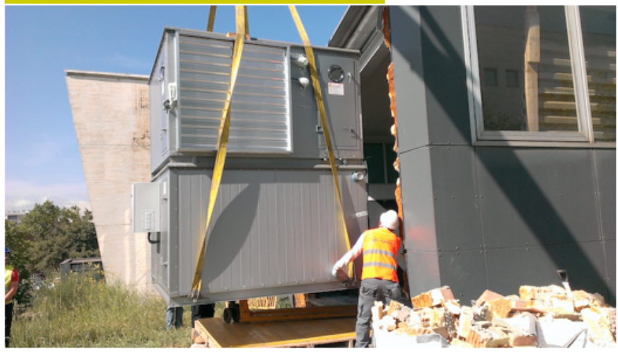
Installation of free-cooling units
