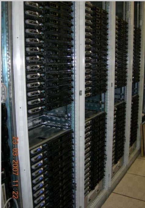
High Level trigger in surface building SDX1
