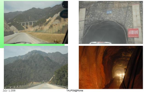
Road and Tunnel
