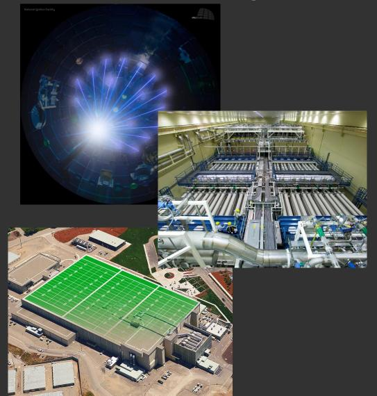
Spec:  $\lambda$ = 0.35mm Total energy (to target) = 2 MJ Pulse length = 20 ns Number of beams = 192 Beam configuration = polar Scheme = Indirect drive
