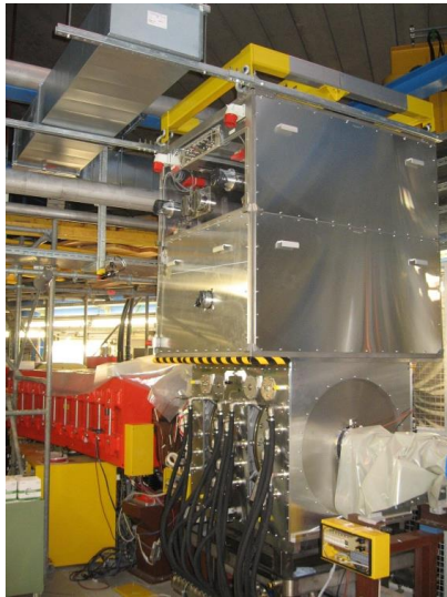
Three new MA acceleration cavities installed (50 kV, h=2)
