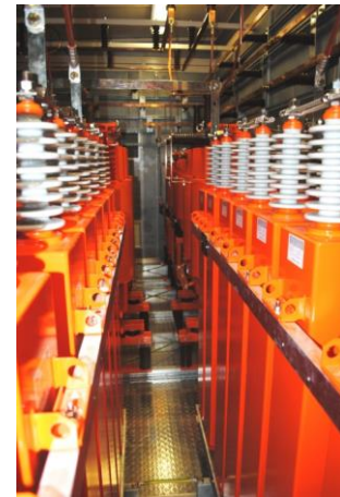
Replacement of main dipole power converter completed (10 T/s, 50 MW)
