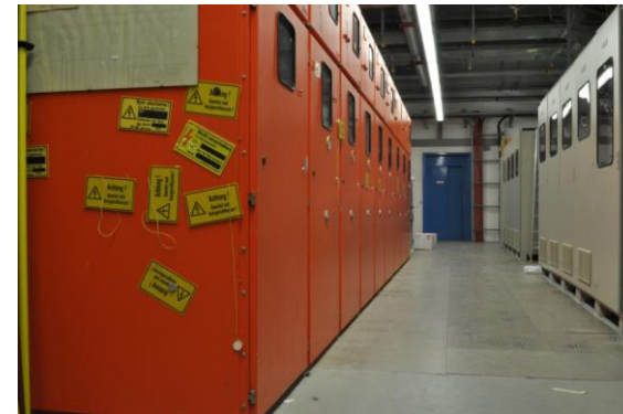
Replacement of main dipole power converter completed (10 T/s, 50 MW)
