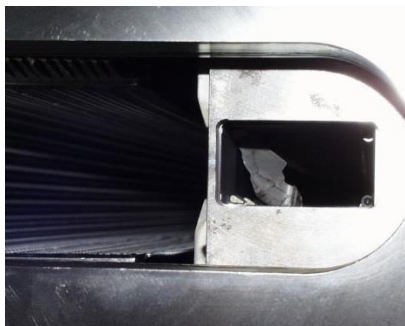
Lamination fatigue failure on PE SMH16
