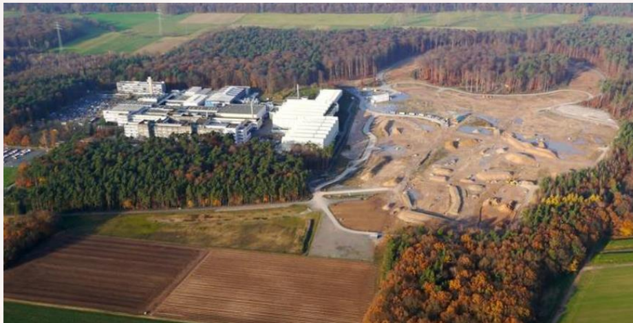
View of construction site
