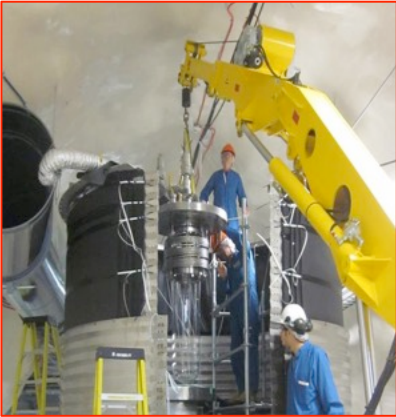
PICO-60 installation in water tank at Snolab
