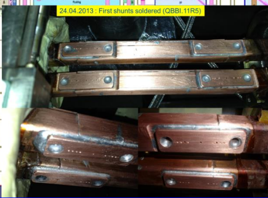
First shunt soldering on 24.04.13
