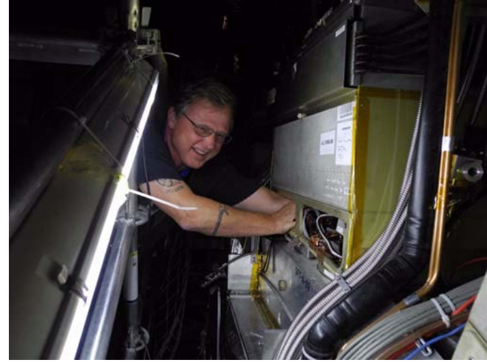
Plugging warm cables into new backplane
