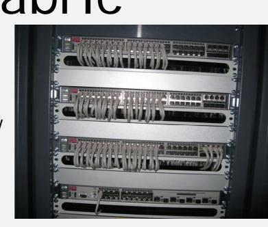
high performance core network (2.4Tb/s switching capacity and designed for fully non-blocking performance) whilst keeping per-port costs low. Using Ethernet as the unique interconnection technology (as opposed to FiberChannel or Infiniband) avoids costly and inefficient translation gateways to connect to the rest of CERN, the experiments and the T1s.
