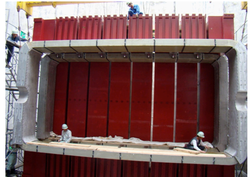
Coils installation
