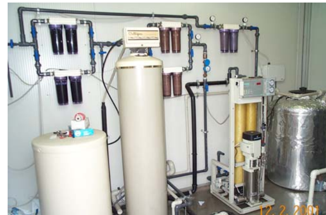
Ultra-pure water system (1200 l/h - 18 M \Omega cm)
