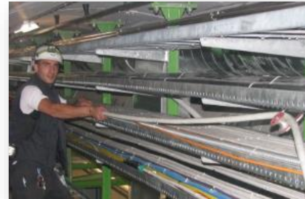
Cabling campaign @P1
