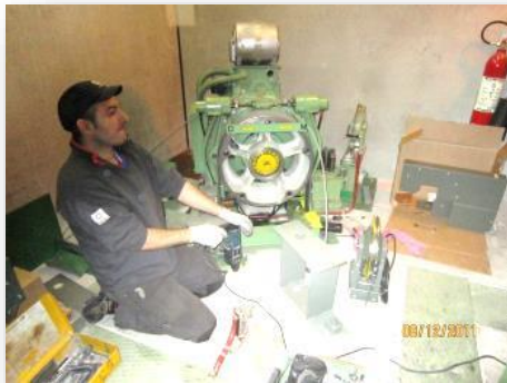
Lift - speed limiting device
