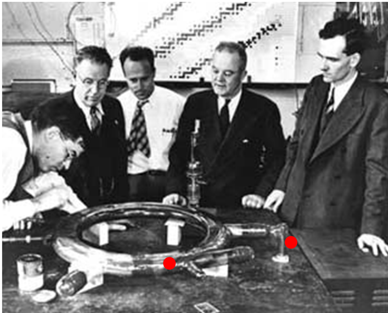
Glass vacuum chamber of the 1947 General Electric Synchrotron Accelerator (70 MeV). Courtesy BNL and ESRF.
