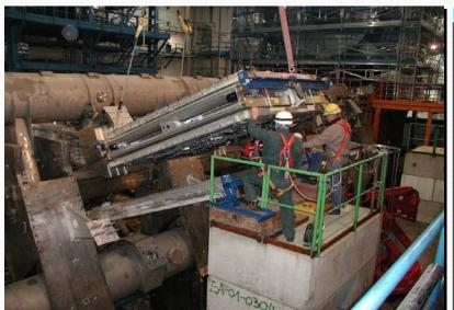
Installation of barrel muon station (40% done)
