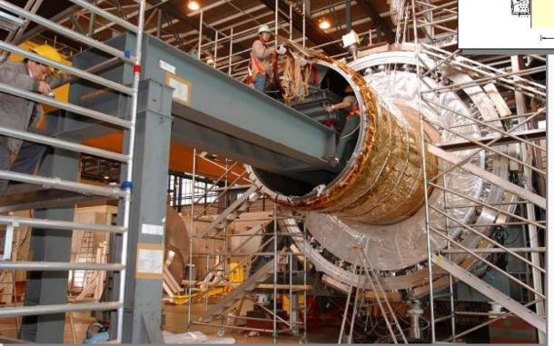
Solenoid has been inserted into the Lar cryostat end Feb 04 and tested at full current (8 kA) during July 04
