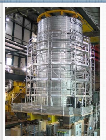
Magnet has been built out of 5 modules, connected and leak-tested.
