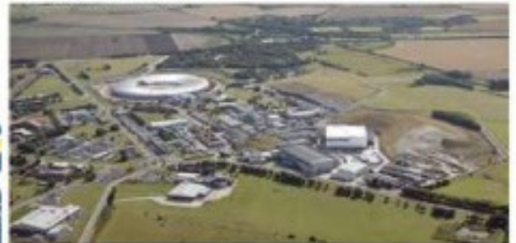
Rutherford Appleton Laboratory Harwell Science and Innovation Campus Didcot, Oxfordshire
