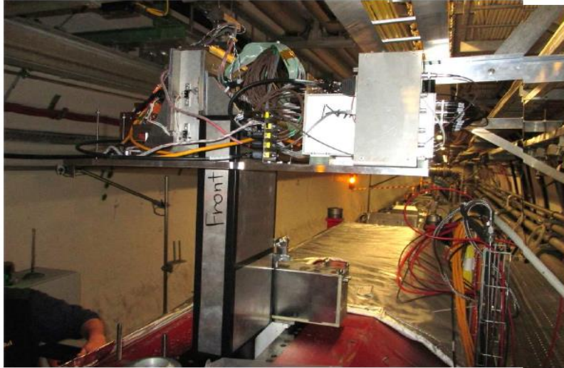
Fig. 9.52: LHCf Arm1 detector and its front-end electronics being installed into the TAN instrumentation slot.
