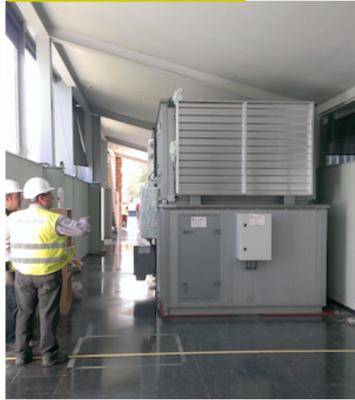
New technical area
