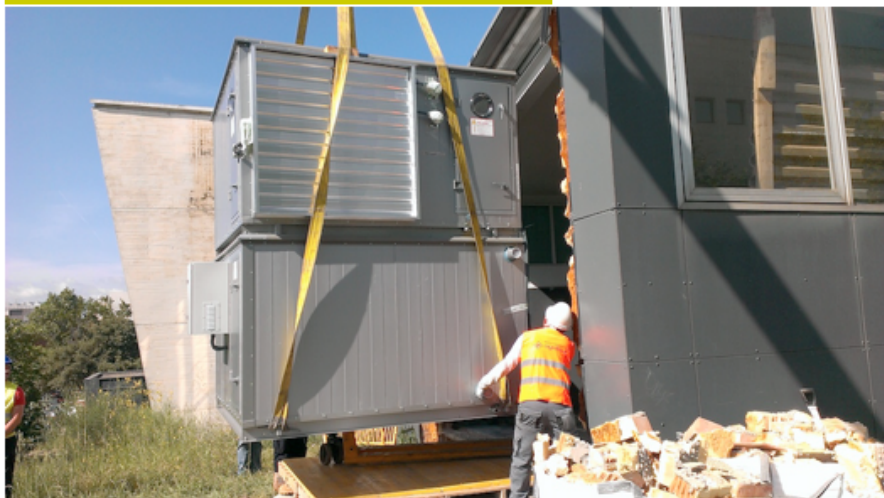
Installation of free-cooling units
