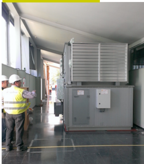
New technical area
