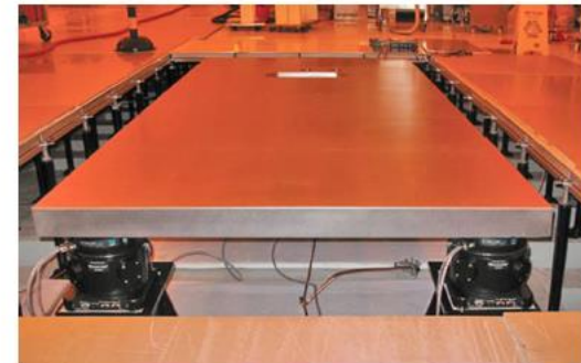
STACIS Isolators supporting a Steel Laminate Platform in a Raised Floor
