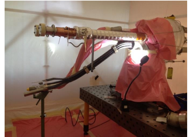
Repair of DFBAK SHM in B112
