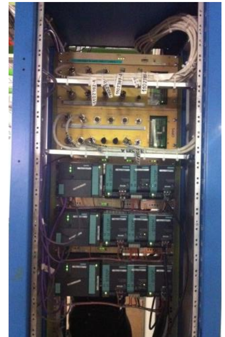
PIC installation in UL16
