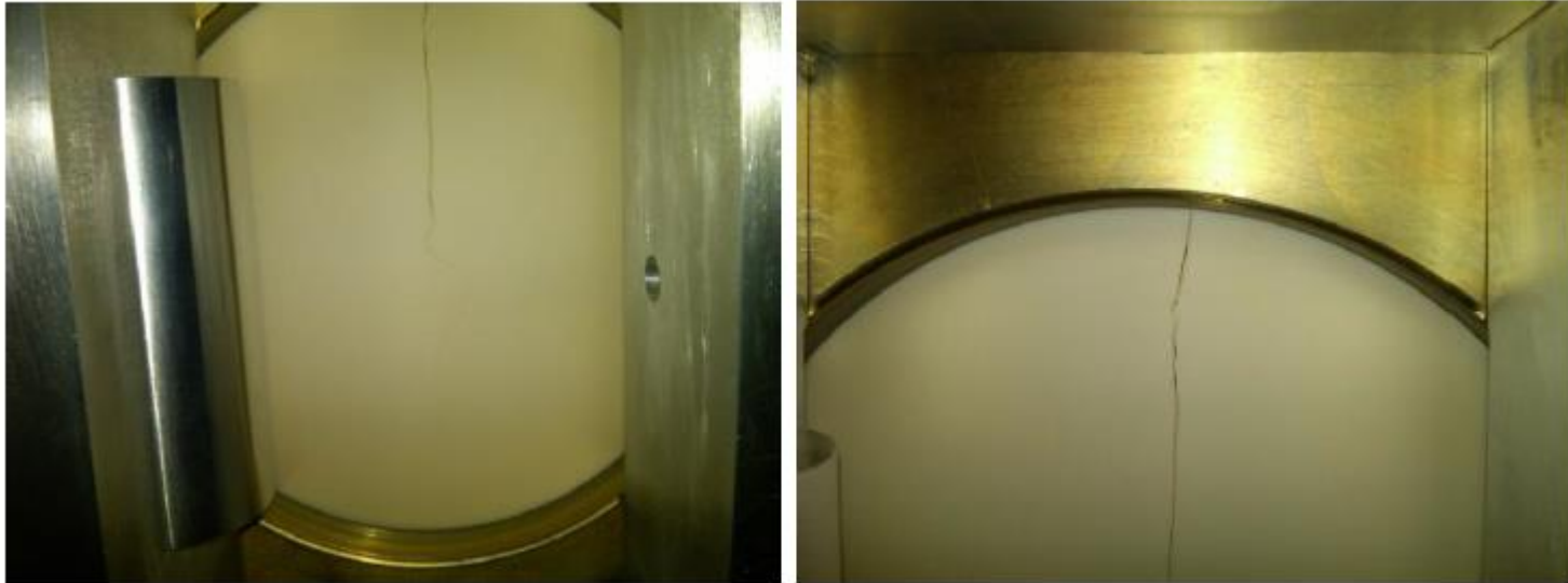
Figure 3 - CCL Window with fracture of ceramic window.
