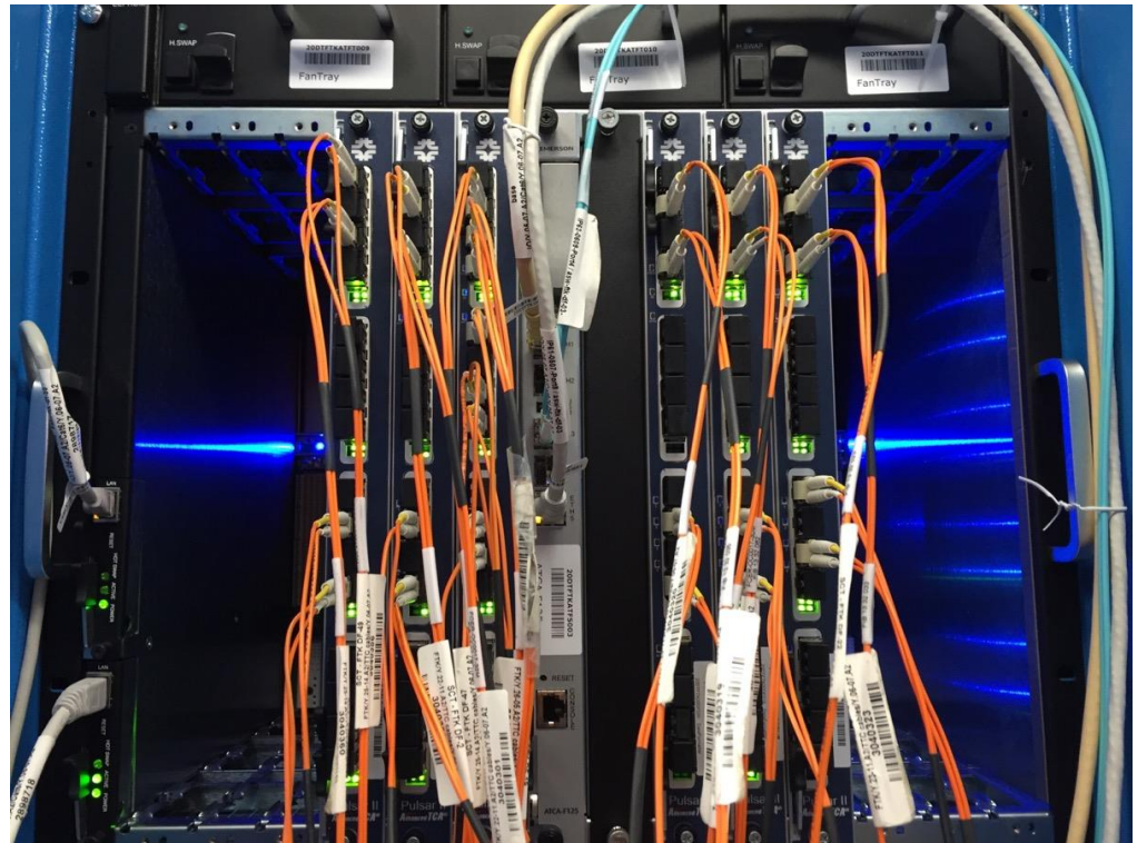
Installed DF and IM boards
