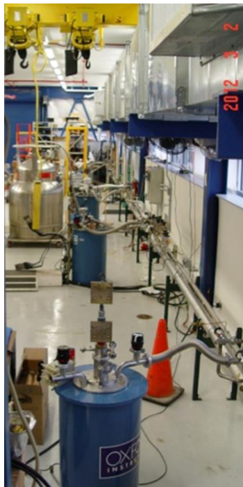
Strand and Cable Lab
