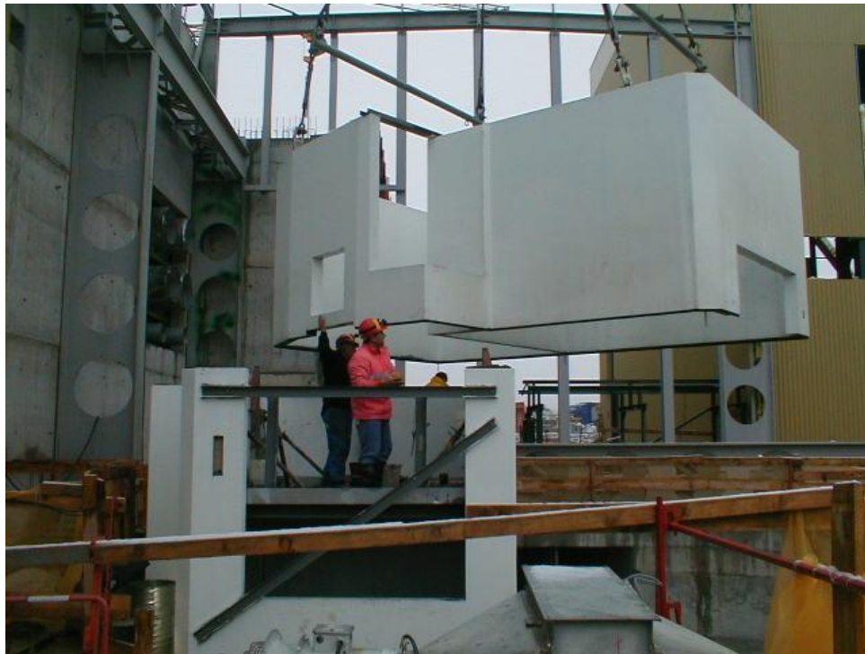
Precast Concrete lift modules in shaft
