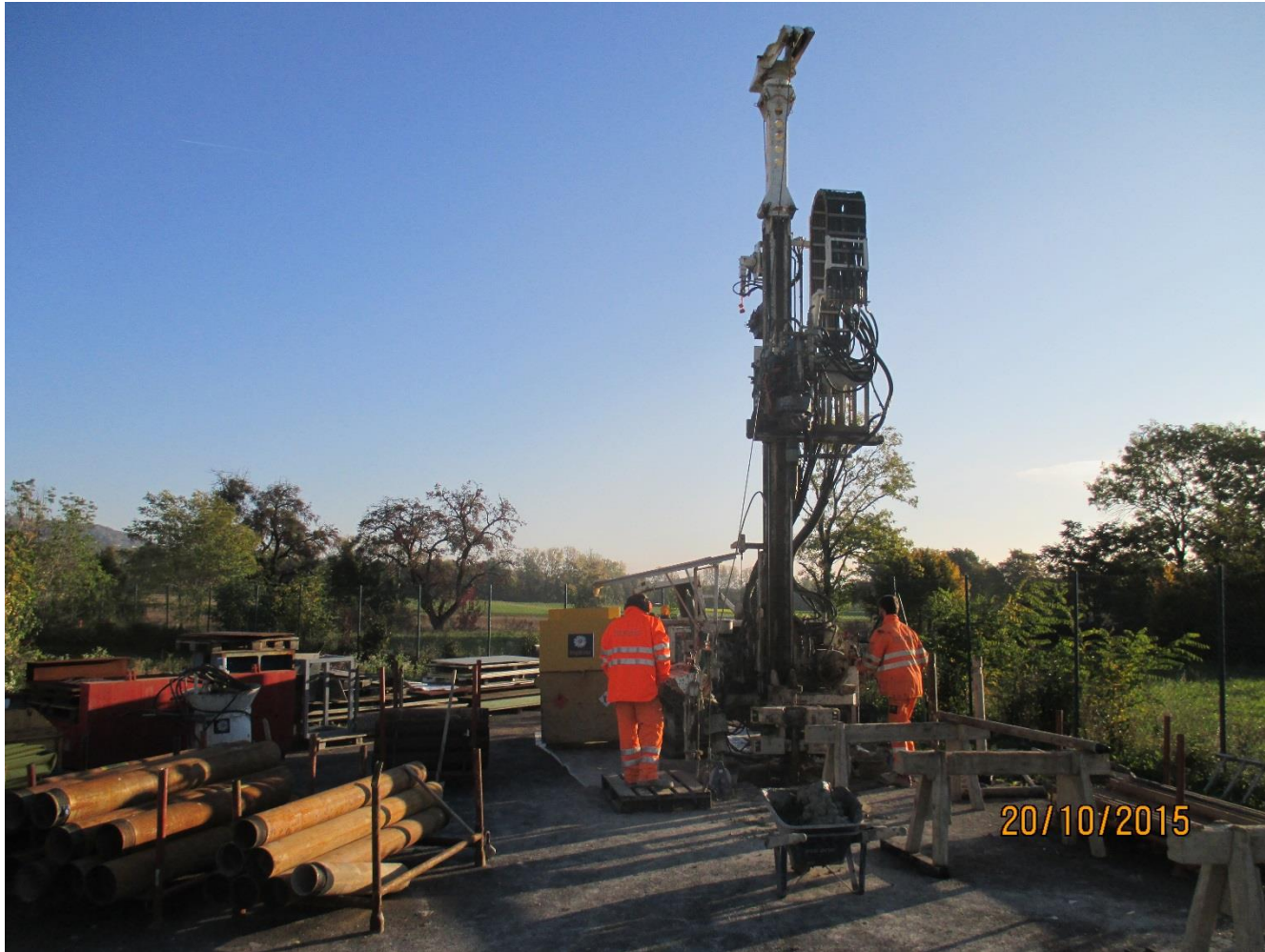
Test drilling for new shaft at LHC Point 5 CMS
