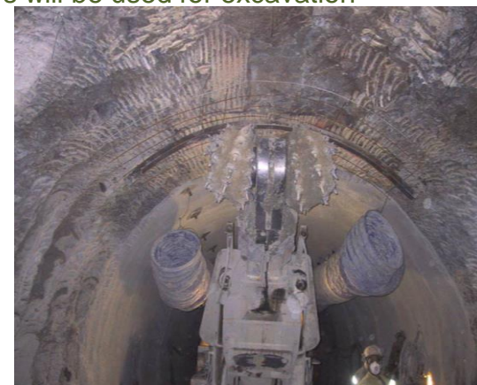
Roadheaders will be used for excavation
